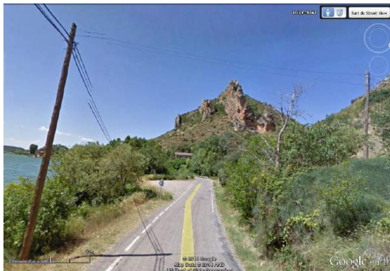
Post with tension cable that crosses the road
